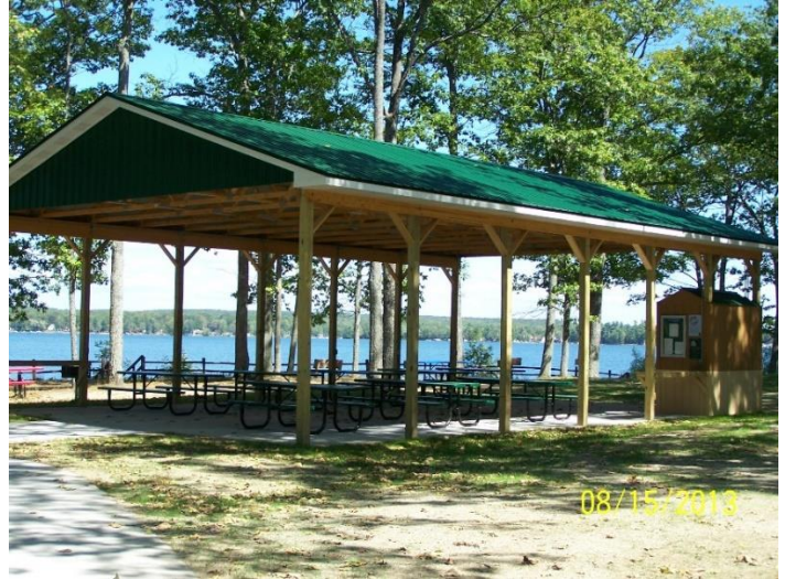
Sands Park Pavilion
